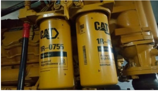
Figure 5. Fuel filter components
