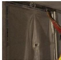
Gambar 5. Pemasangan *engineering door* dilapangan
